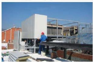
The ground on which the acoustic cabin or enclosures has to be mounted should be totally flat. In the case of acoustic barriers, a perimeter leveling concrete band has to be built. Panels should be installed vertically and assembled using the dovetail system. With the help of the special profile, PF80 (see diagram below) proceed to assemble the 450 mm wide modulated panels. Special width size panels can be manufactured on request according to requirements needs.
